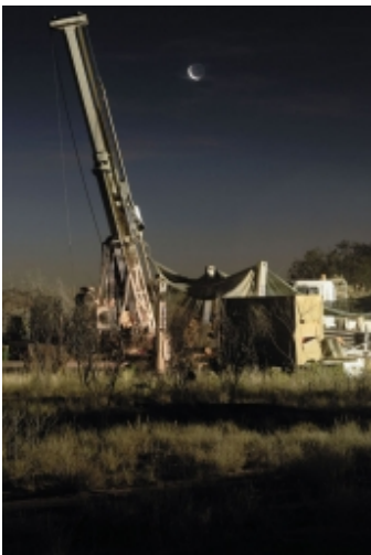
Drilling at Rover near Tennant Creek.
