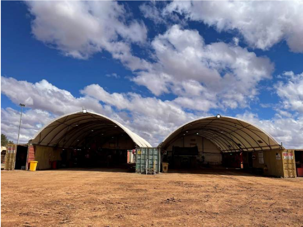
Figure 18-2 Fortnum underground workshop - Source: Westgold.
