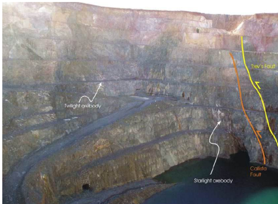
Figure 16-3 Major faults in Starlight Pit. Source: Westgold.
