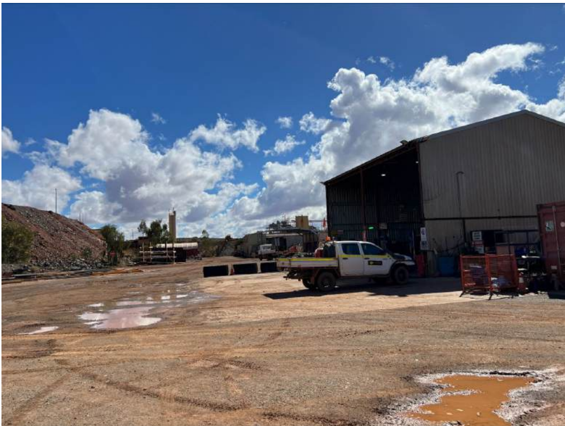
Figure 18-3 Fortnum light vehicle workshops - Source: Westgold.
