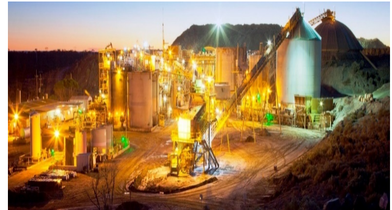
1.2 million tpa CIL Plant
