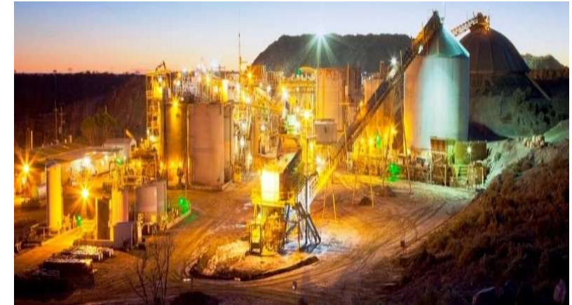
1.2 million tpa CIL Plant
