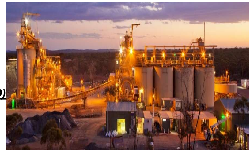
1.3 million tpa CIL Plant
