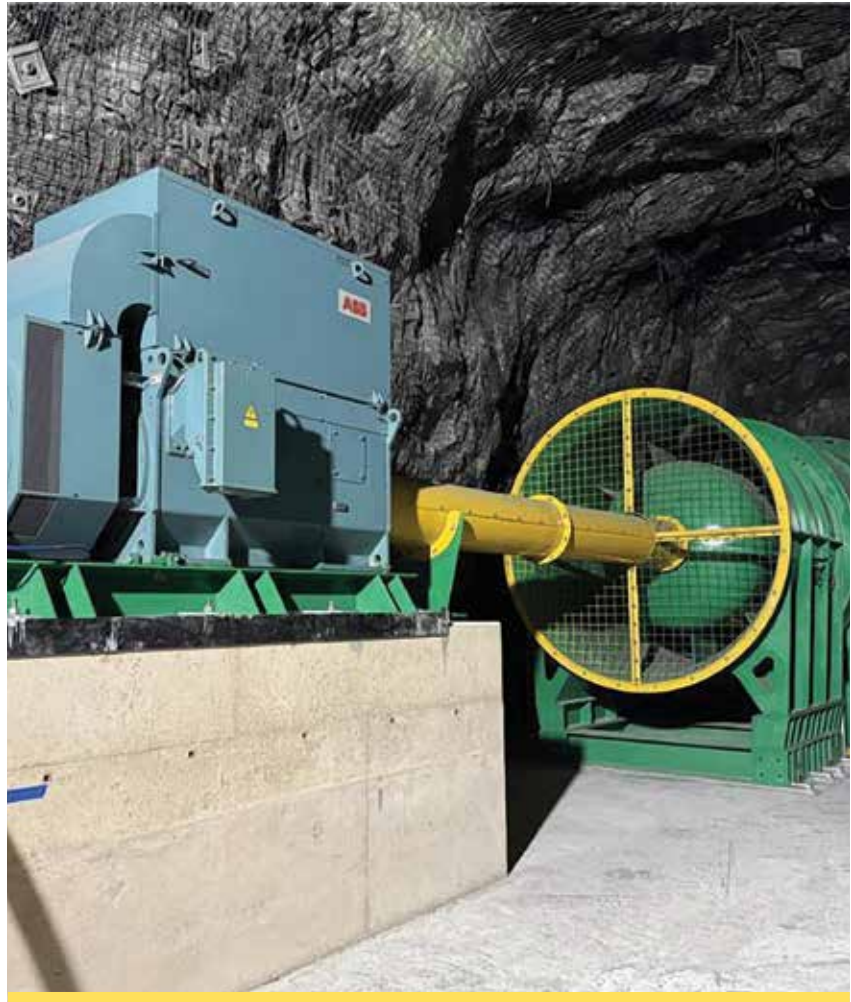
Beta Hunt Infrastructure Upgrade
